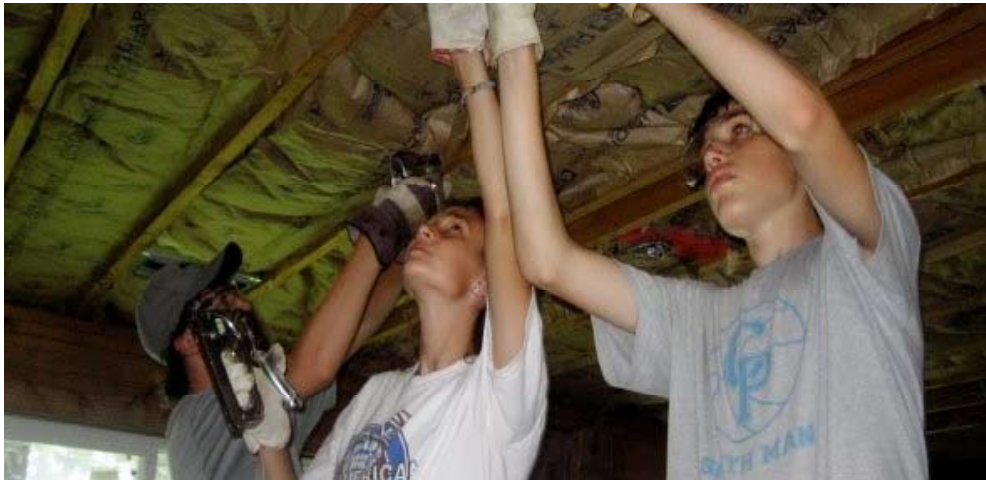
Amanda Haltmaier (V) repairs a devastated home.
