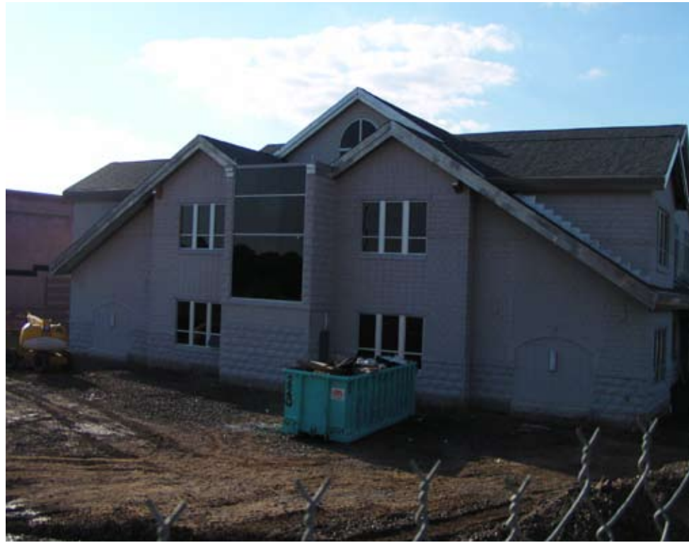
The new Middle School is adjacent to the current structure.
